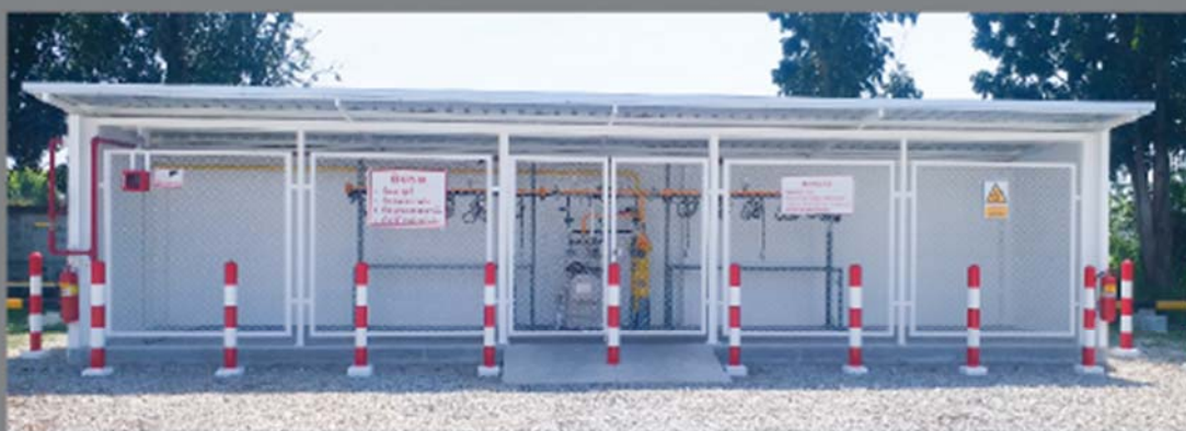
YANAGAWA AT EASTERN SEABOARD INDUSTRIAL ESTATE (RAYONG)
