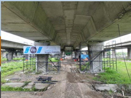
Bearing Replacement: Motorway No.9
