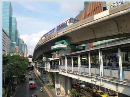
Bearing Replacement: BTS Saladaeng
