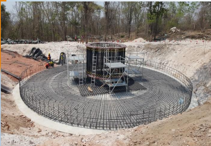
▲ One of the turbine foundation formwork.
