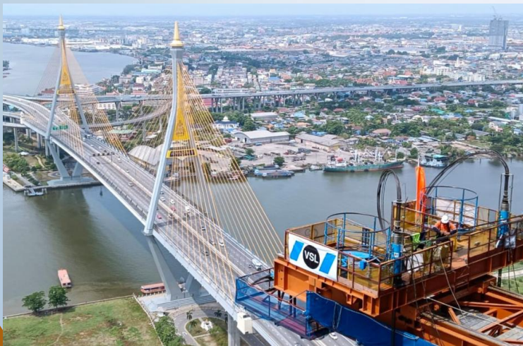
▲ The site is located nearby our previous mega project, the Industrial Ring Road Bridge (Bhumibol Bridge)
