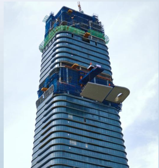
▲ Lifting of truss elements for sky lounge
