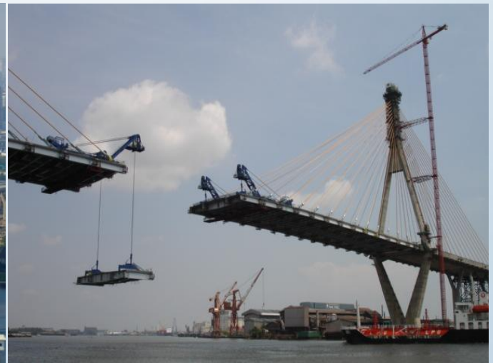
▲ Bridge deck erection and supply and installation of stay cable.
