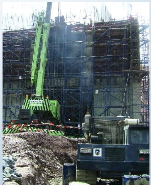
▲ During construction, it enables for ground stability.
