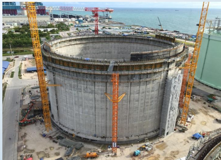
▲ Tank under construction
