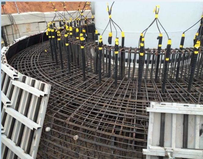
▲ Repair work in process.
