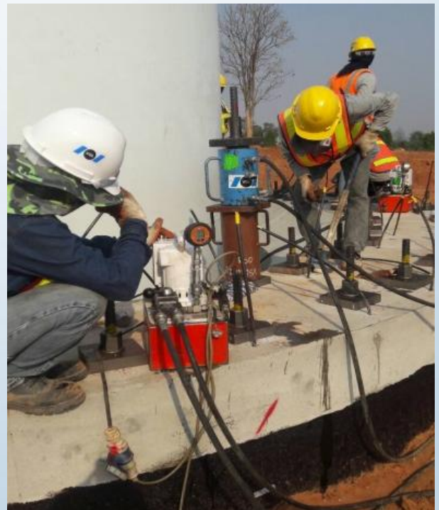
▲ Coring existing wind turbines foundation for PT bar system.
