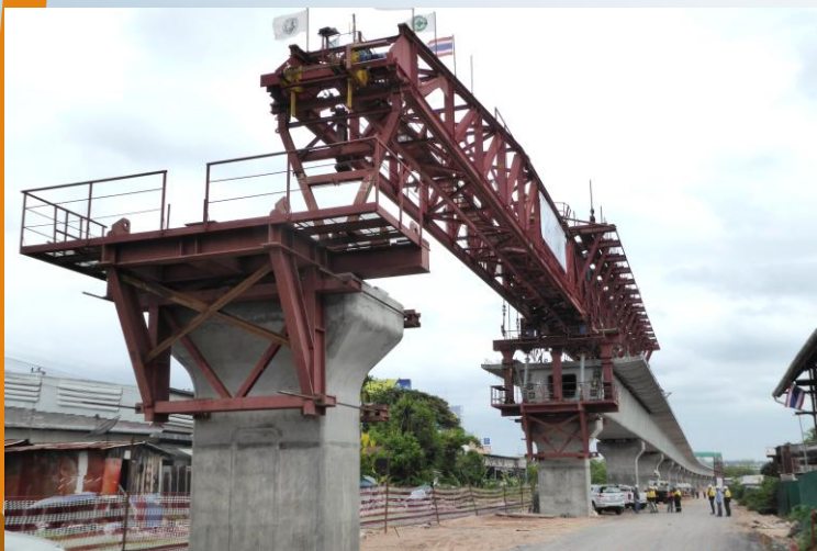
▲ VSL launching gantry
