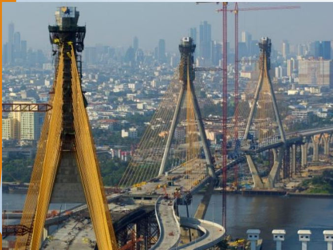
▲ Stay cable composite bridge across Chao Phraya River with bustling 7 traffic lanes.
