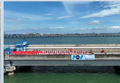
KSSP Jetty Repair with External PT
